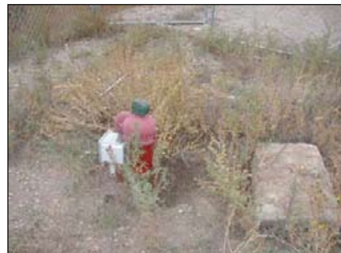
Another example of an unprotected wellhead.
