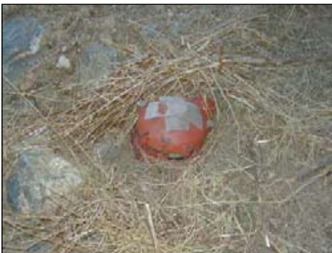
Example of an unprotected wellhead.
