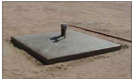
Example of a properly protected wellhead.
