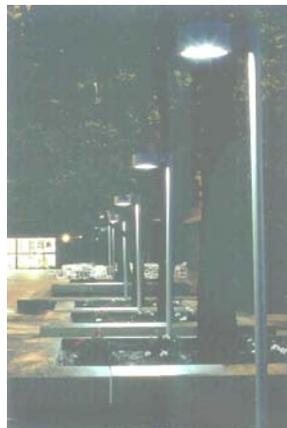
**Figure 3. Minimized direct glare with IESNA full cutoff luminaires.**
