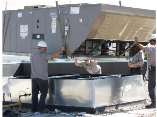
*The upgrades to the City of Lafayette's facilities included new energy efficient roof top units for heating and cooling*
