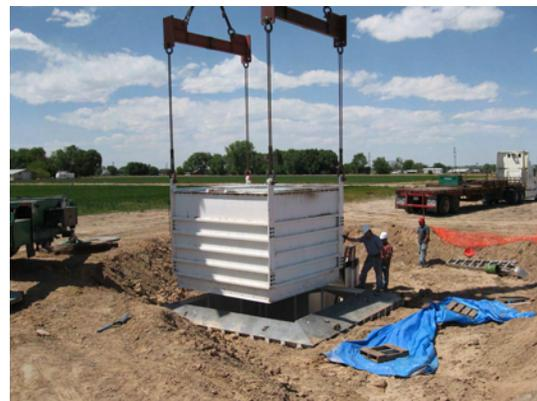
**Figure 4.** The inner tank plus soil being lowered inside the containment tank. Photo by Michael Bartolo.
