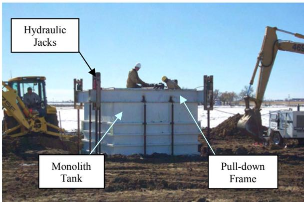
**Figure 1.** The inner tank being pushed into the ground to acquire the soil monolith. Photo by Dale Straw of DWR.
