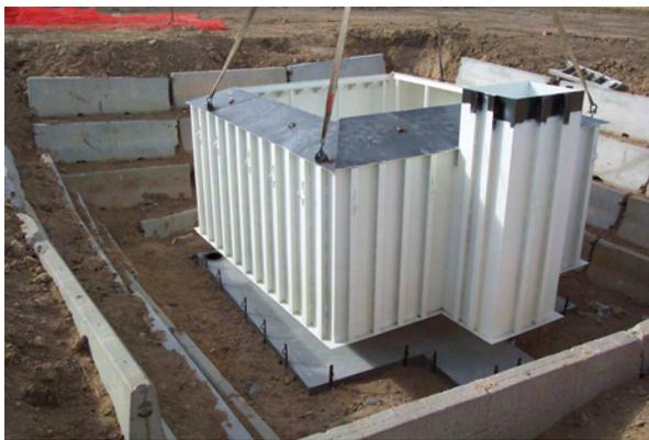
**Figure 3.** The outer tank being lowered into position. The concrete slabs were used to hold the soil in place. They were taken out before re-filling the empty space around the outer tank. Photo by Dale Straw of DWR.
