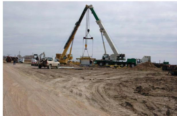
**Figure 2.** The inner tank plus soil being lifted off the ground prior to moving it to its permanent location. Photo by Abdel Berrada.
