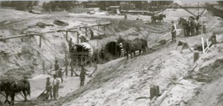
*Teams of horses were the only heavy equipment available to help excavate early canals, ditches and reservoirs across the West. Water delivery pipelines (above) originally were made of wood, and had to be replaced often.*
