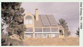
PV systems operate almost anywhere. The system output varies less than 15% from the best solar resource in the state to the worst. Most days in Colorado are sunny, but even on cloudy days PV systems produce about 25% of their output.
